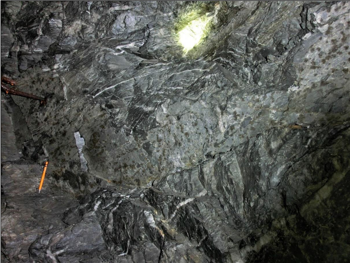
Figure 5.3: Photo of the rock mass in the niche at chainage 255 of the R1. The rock is more fine-grained and heterogeneous than at chainage 430, with more frequent quartz bands and folds. Pen for scale.
