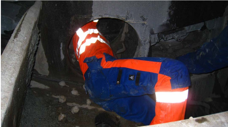
Figure 4.1: Inspection hole at the ARM Project.
