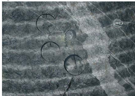
Figure 4.4: A) Core drilling into the face of the Nedre Røssåga headrace tunnel. B) Picture showing a typical sampling pattern.
