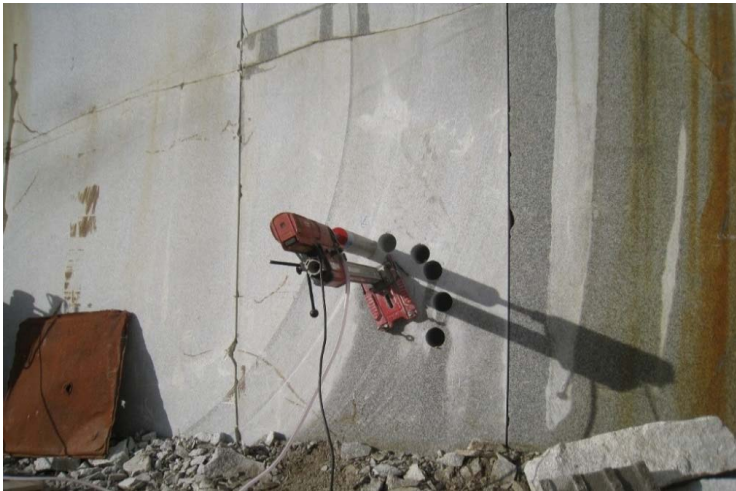
Figure 4.8: Core drilling at a vertical wall at the Trondhjemite quarry.
