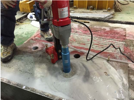
Figure 4.10: Core drilling after testing. Note that the core drilling were performed from the bottom of the specimen (photo: Yongbeom Seo).
