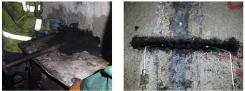
Figure 3. Installation of flatjack in the slot (left) and connection to the pressure measuring transducer (right).
