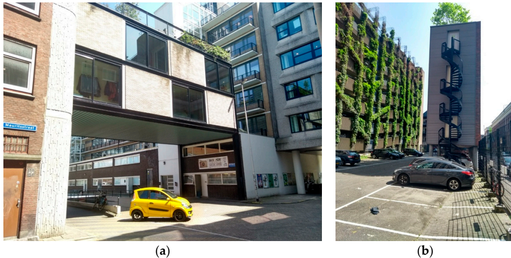
Figure 8. (a) Mauritsstraat, Cool, infill densification strategy, by Kühne en Co. (Rotterdam, The Netherlands); (b) Boomgaardstraat, Cool, Kühne en Co. (photos by Nico Tillie).
