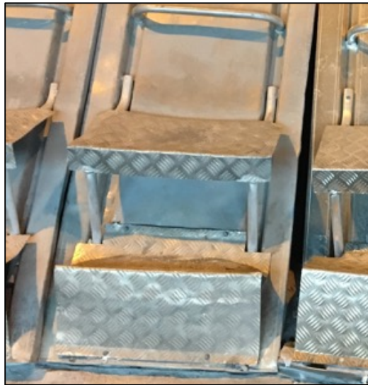
Figure 6.5: A pot cover with moderate denting damages on both lower and upper stepping plate.
