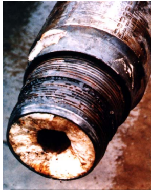
Figure 2.2: Scale crystals in pipe (Mackay, 2008)
