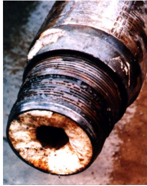
Figure 2.2: Scale crystals in pipe (Mackay, 2008)
