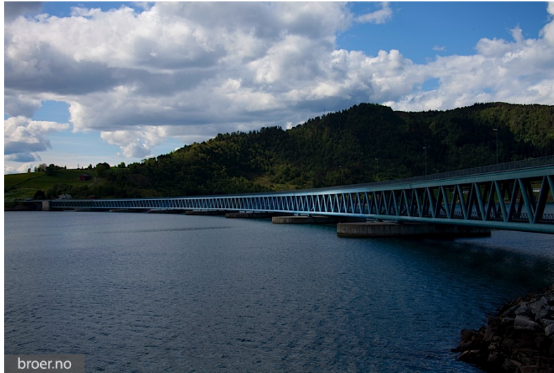
Figure 2.4: The Bergsøysund Bridge, illustration (broer.no, 2018a)
