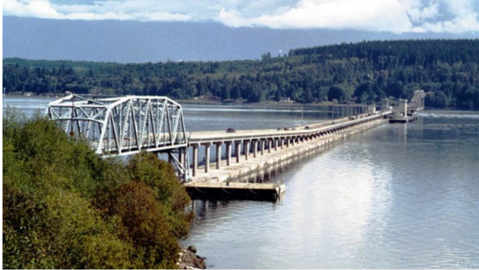
Figure 2.6: Hood Canal Bridge, illustration (Structurae, 2017)
