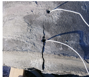
(b) Drilled holes (pipe IV)
