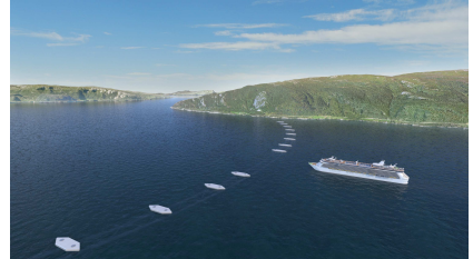
Figure 3.6: Visualization of a ship passing over a pontoon anchored SFT. Credit: NPRA.
