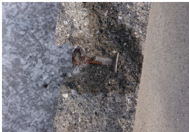
(a) Lifting point (pipe X)
