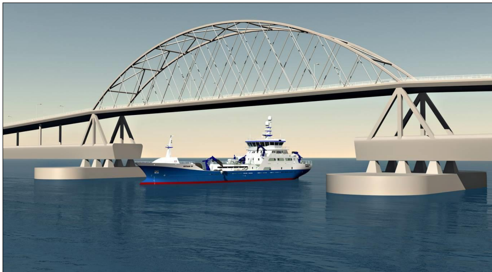
Figure 1-1: Illustration of a floating (pontoon) bridge (NPRA, 2012)
