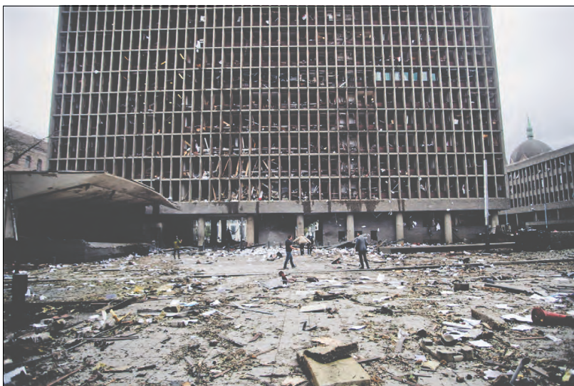
Figure 1.1: Executive Government Building after the terrorist attack 22 nd of July 2011 [1].
