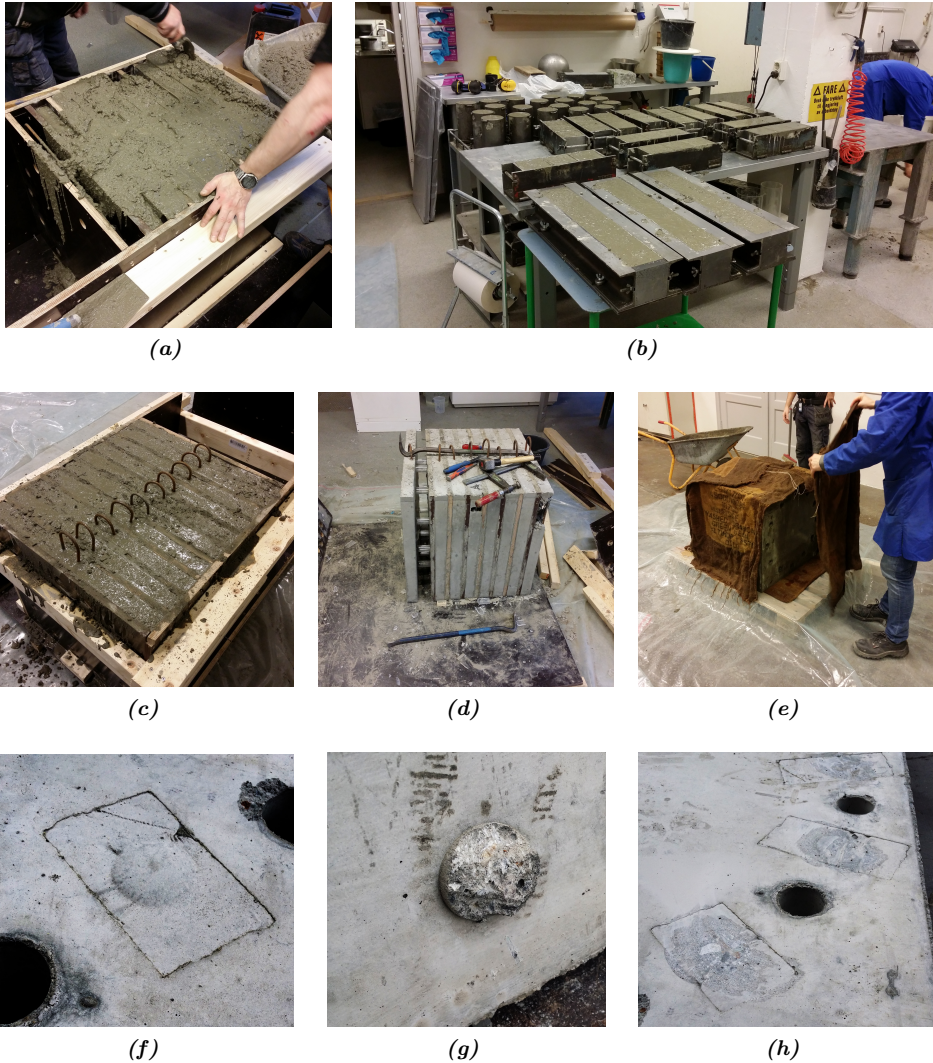
Figure 5.5: Filling the plate formwork (a) and filled material test specimen moulds (b). The creation of concrete plates; fresh concrete in (c), disassembling the formwork (d) and sealing the plates in soaked cloth and plastic (e). Defects in the concrete plates due to (f) bulging of tape covering mistakenly drilled holes and (g) due to missing tape. The plate after grinding is shown in (h).
