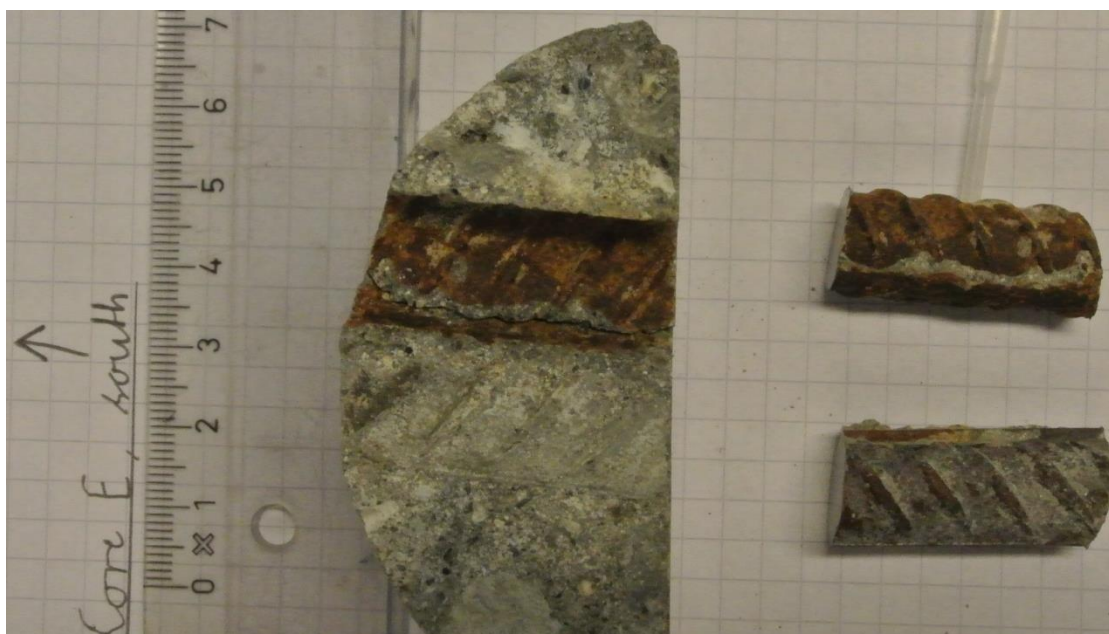
Figure 6.5 Excavating the reinforcement from core E, Moholt Bridge
