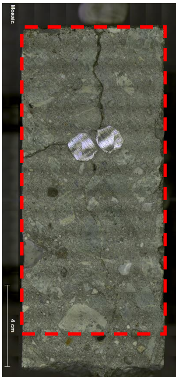
Figure 5.8 Mosaic picture of core E, Moholt Bridge. Exposed concrete surface is on the top.
