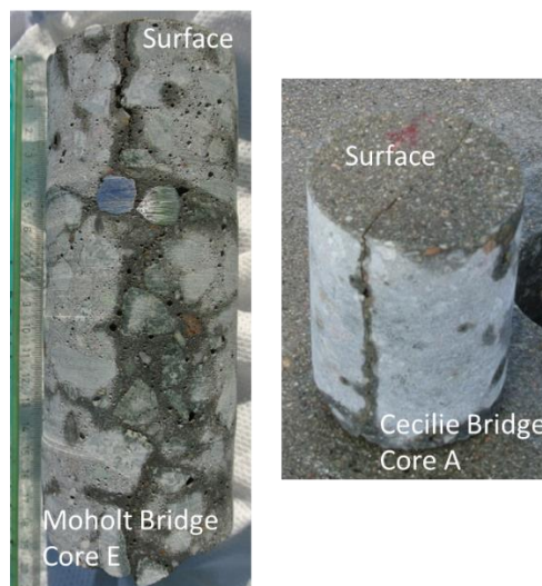
Figure 10.15: Concrete cores E and A extracted from Moholt Bridge (Left; Crack width 0.55 mm, cover 50 mm) and Cecilie Bridge (right; Crack width 0.45 mm). Picture: Andreas Rygg
