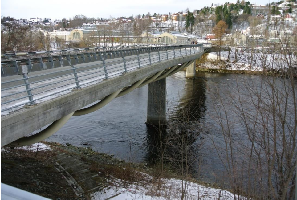
Figure 3.6 A overview of Cecilie Bridge. Note the curved outer edge next to the pedestrian lane.
