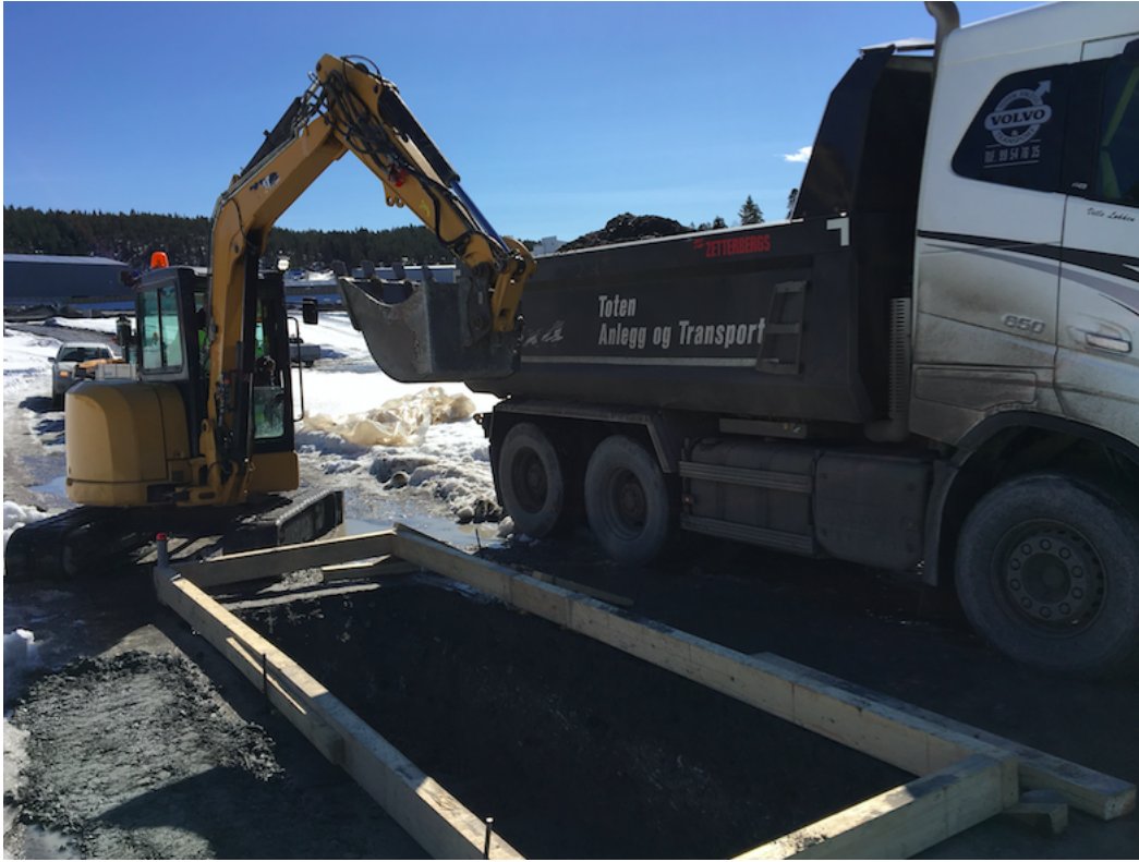
Figure 3.16 – Excavation of test pit
