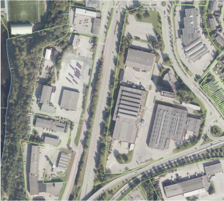
Figure 4.8: The Siemens lot today. Satelite view by Trondheim Municipality
