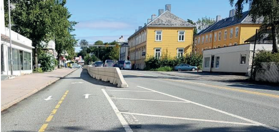
Figure 16. The intervention in Innherredsveien, Trondheim used two forms of separation: painted horizontal lane markings and concrete barriers (photo: pbb/Mapillary 19 , licensed under CC BY-SA 4.0 20 ).
