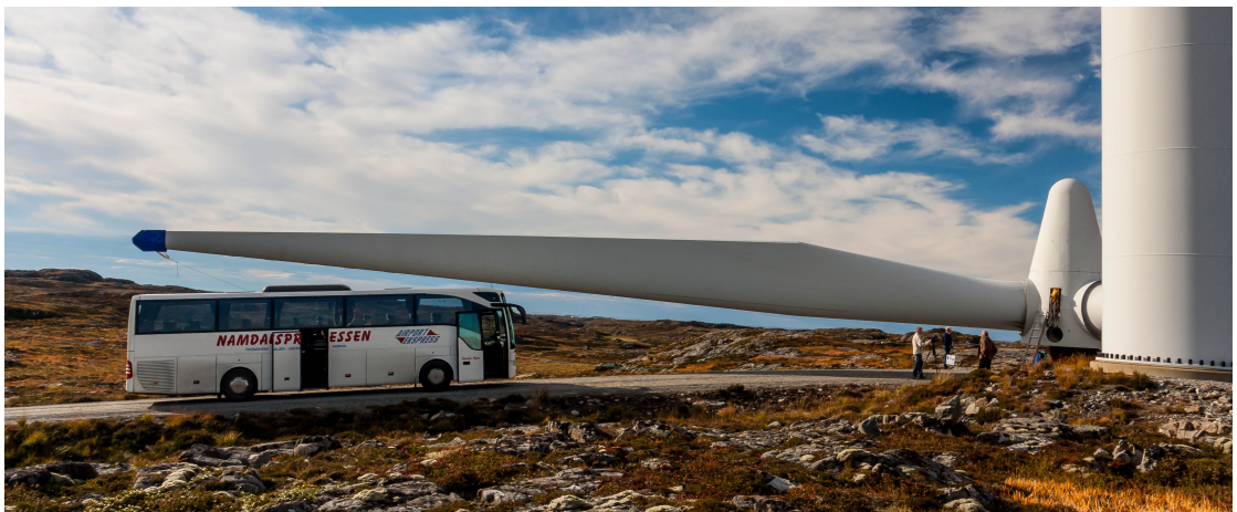
Figure 1.2: Comparison between a 2.3MW turbine blade from Smøla wind farm and a bus.
