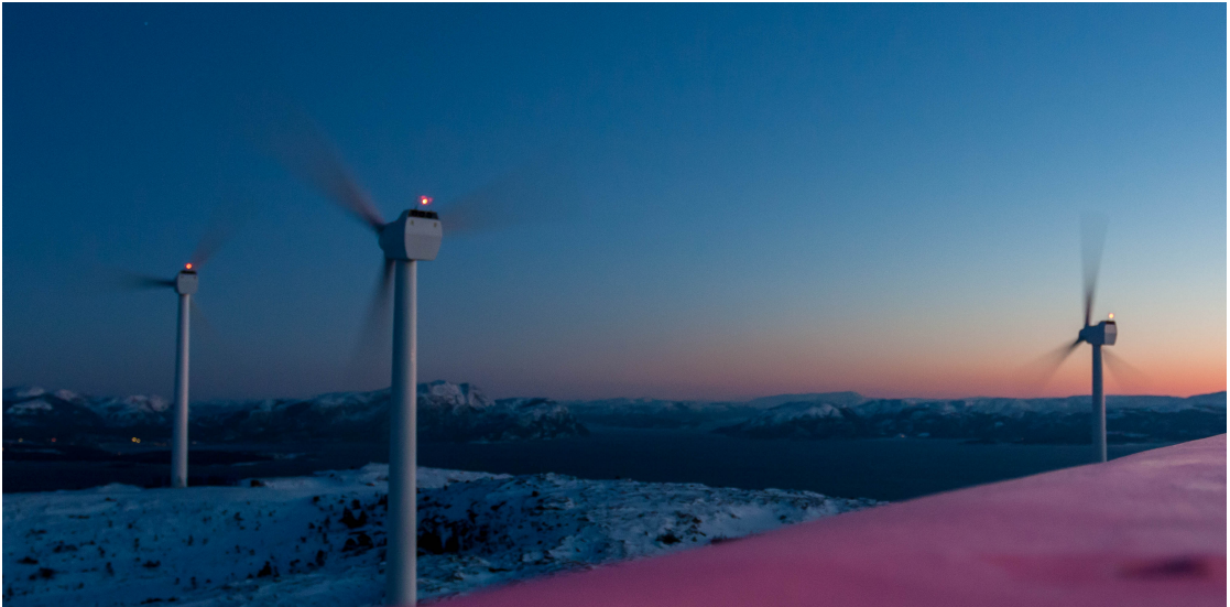
Figure 1.3: View from the top of a wind turbine at Hundhammerfjellet wind farm.
