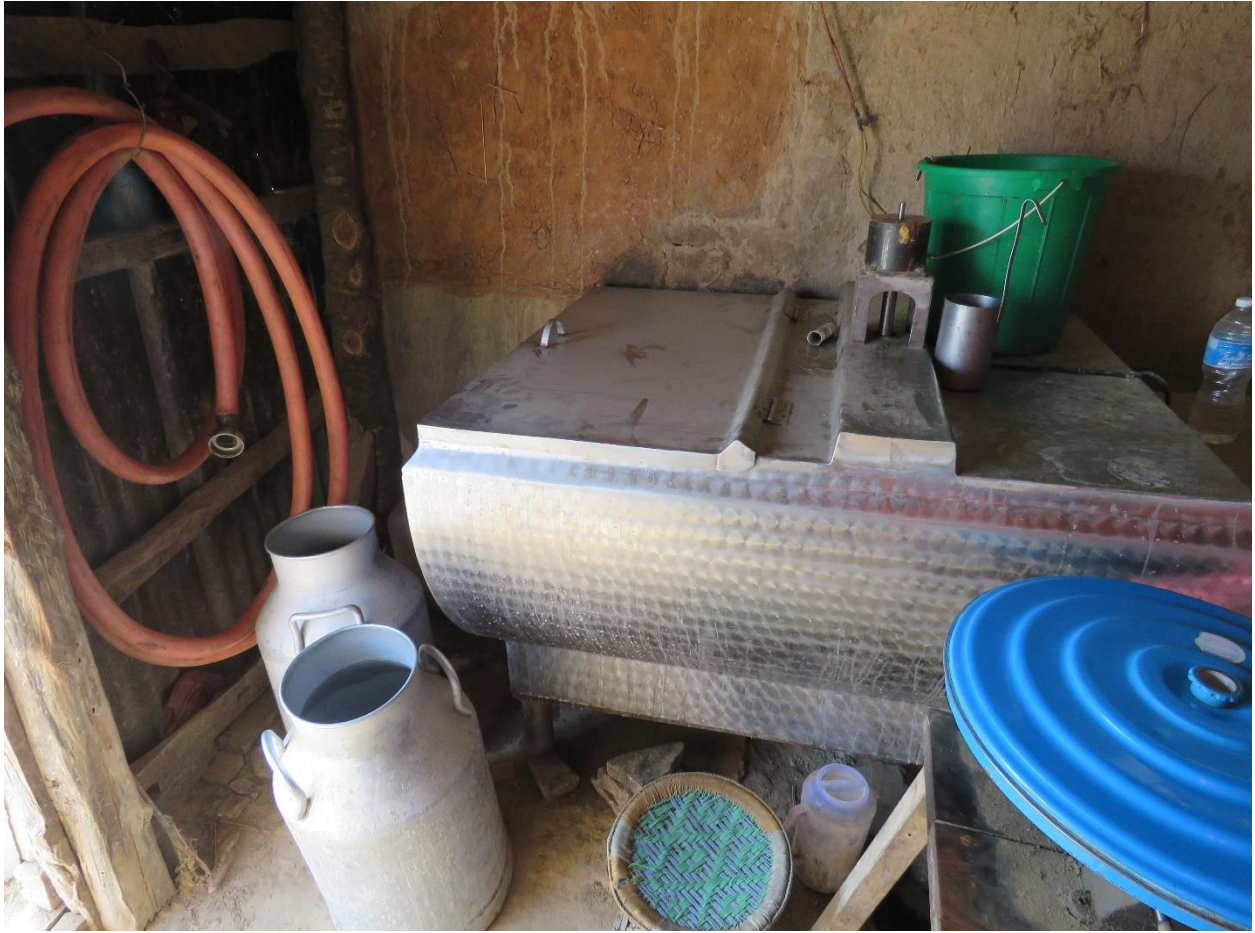
Inside the community milk collection centre, with 20 litre milk jugs on the floor and milk collection tank in the centre.
