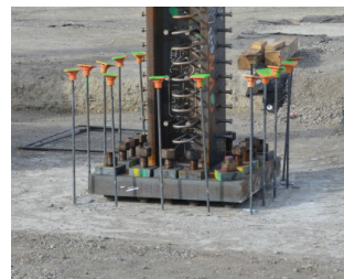
Rebar Caps (Source: Iris D. Tommelein)
