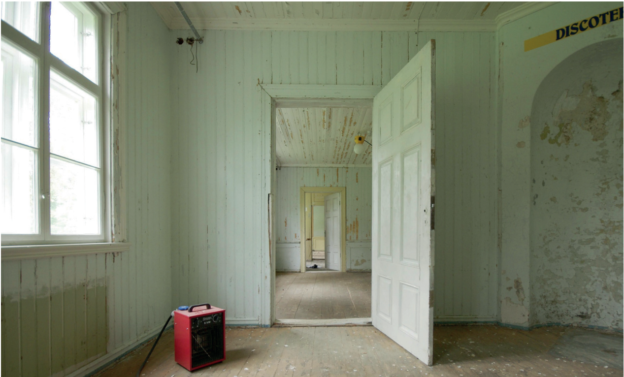
Photo 1. Typical room on ground floor
