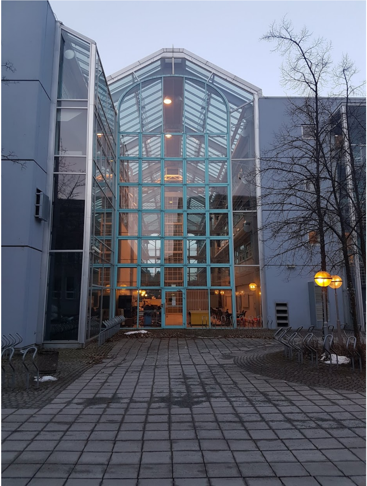
Figure 4.9: Outside view of the atrium Koopen is located in. Note the large glass surfaces.
