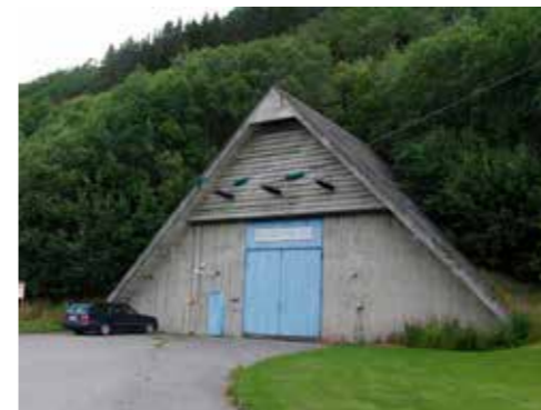
Entrance to Ylja power plant
