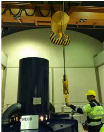
A crane used as a fixed reference to demonstrate the vibrations during a visit in October 2017
