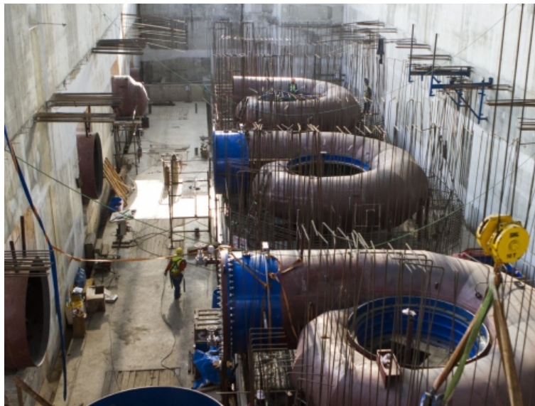
Figure 3.1.3: Three major Francis turbines under construction. [41]
