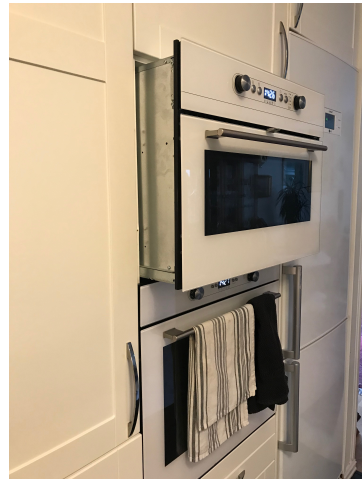
(a) Smart meter with EcoMonitor connected. (b) Removing microwave and oven to install smart plugs.
