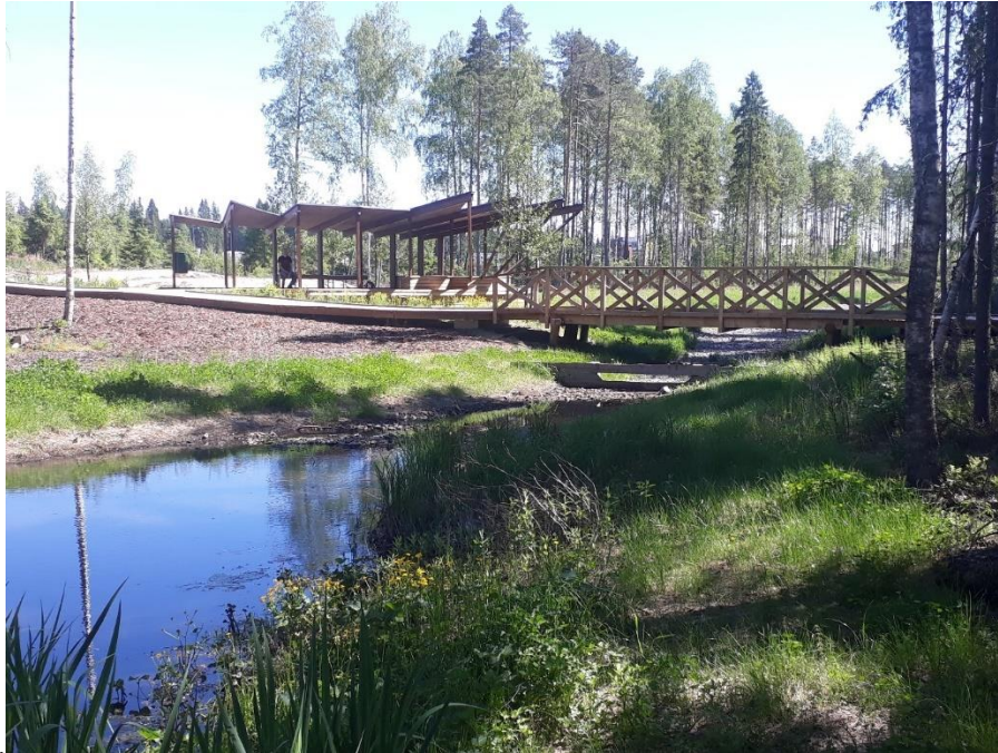
Figure 29: Stormwater is conveyed partly daylighted and partly underground by filtering through crushed stone. Right before the wooden bridge, the water is led underground. In heavy runoff events, water will rise up of the crushed stone and also be conveyed on the surface. The municipality arranged a design competition and co-created a roofed picnic sitting area together with the winning design company (H2PM1).
