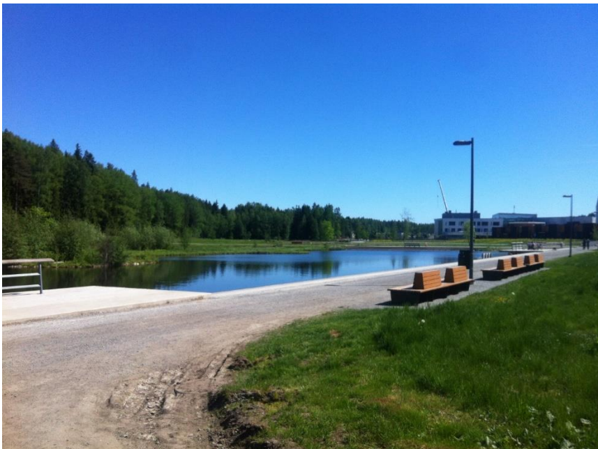
Figure 24: The Central Dam in Vuores Central Park in the end of May 2018. Inhabitants were happy and proud of the park in the flourishing summer months. Stormwater from the housing area are collected in grassed basins along the dam, and the stormwater filters into the dam.
