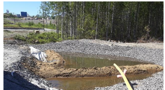
Figure 26: A high groundwater table gives muddy waters during construction. The water is treated in contemporary facilities by filtering through sand and fiber cloth, and pumped to the already constructed NBS for further treatment before release to the vulnerable small lake recipient (H2PM1).
