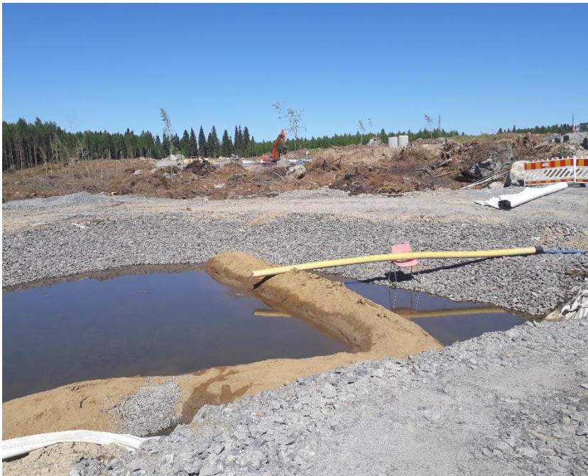
Figure 26: A high groundwater table gives muddy waters during construction. The water is treated in contemporary facilities by filtering through sand and fiber cloth, and pumped to the already constructed NBS for further treatment before release to the vulnerable small lake recipient (H2PM1).
