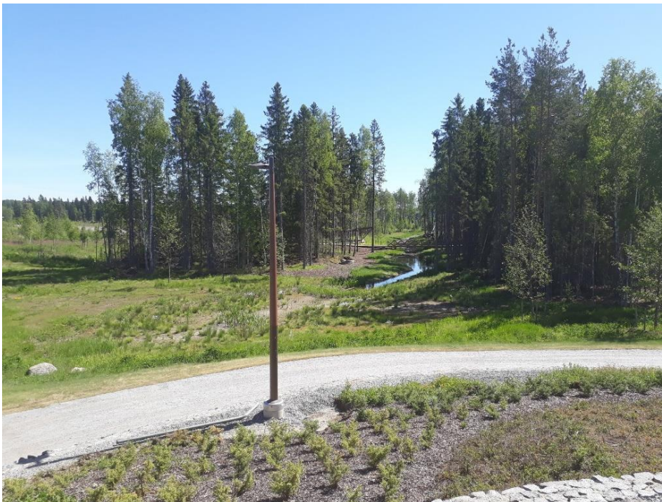
Figure 28: The stormwater area seen from the Tervaslammen bridge
