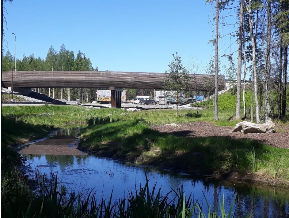
Figure 27: Area collecting stormwater runoff from surrounding development plots. In extreme events, the area will also receive runoff from Tervaslammenpuisto from under the Tervaslammen bridge (H2PM1).
