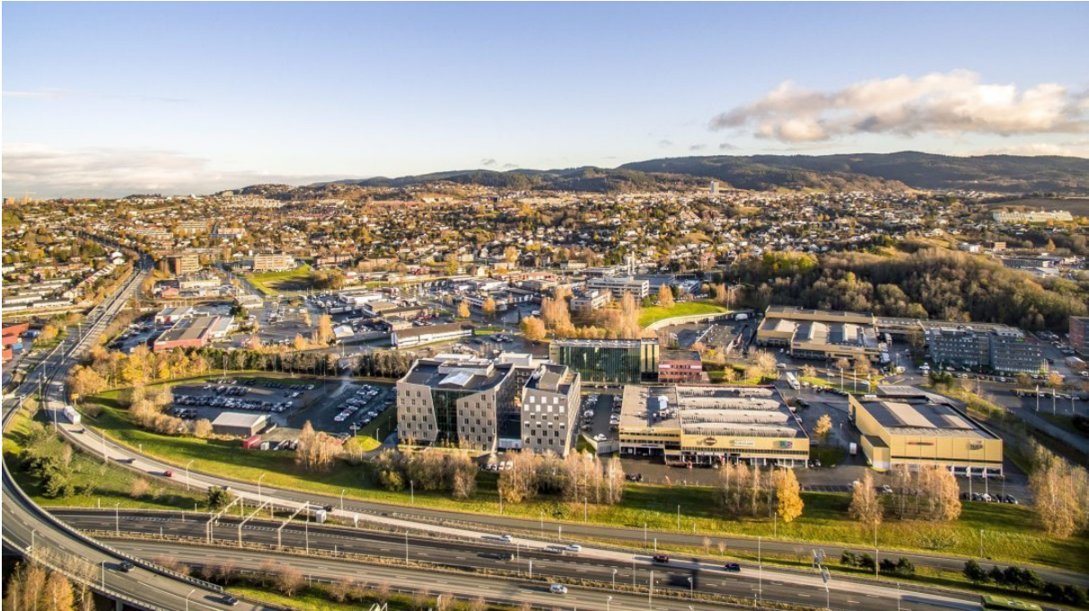
Figure 10. Aerial view of Sluppen, from east. Photo: R. Kjeldsberg
