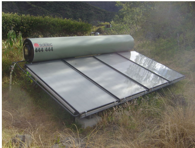
Figure 2.4: Solelec integral direct-gain solar heater
