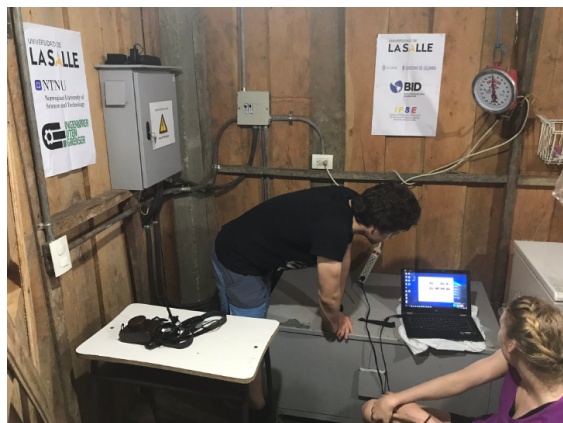
Fig. 4. Installation Process in the refrigeration center
