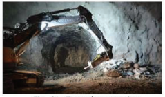
Fig. 2a. Tunnel excavation
