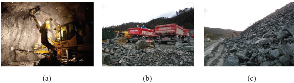
Figure 2 Tunnelling operations: blasting (a), transporting (b) and stockpiling (c) rocks
