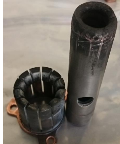
Fig. 3. Eroded contact surfaces after interruption of the rated short circuit current: Moving Contact (left), and Fixed Contact (right).
