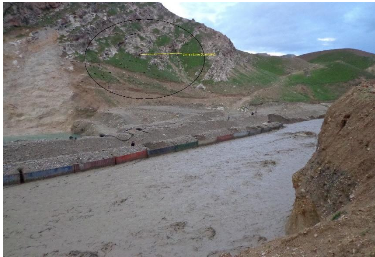
Figure-1. Almar Dam site. Limestone dissolution cavities at the surface
