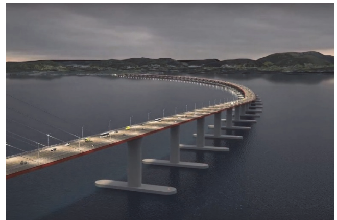
Figure 1 Concept illustration of the end-anchored floating bridge crossing the Bjørnefjord; (Statens vegvesen, 2017)
