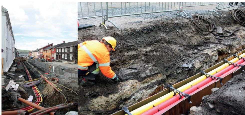
Figure 2.2. Watching brief excavations in Bergmannsgata, Røros in 2013. 138
