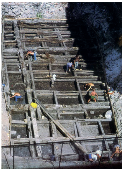
Figure 2.1. Excavations of caisson foundations at Revierstredet 5-7, Oslo. Photo: Riksantikvaren
