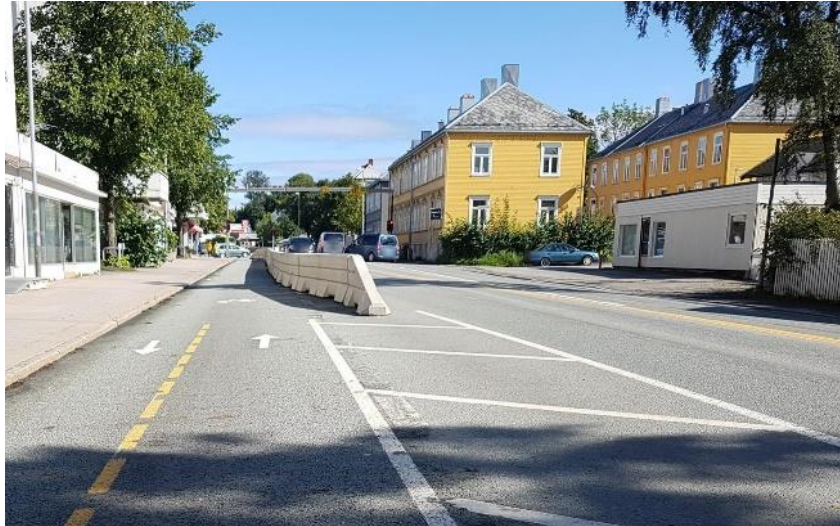
Figure 2. The Complete Streets trial project used two forms of separation: painted horizontal lane markings and concrete barriers [27].
