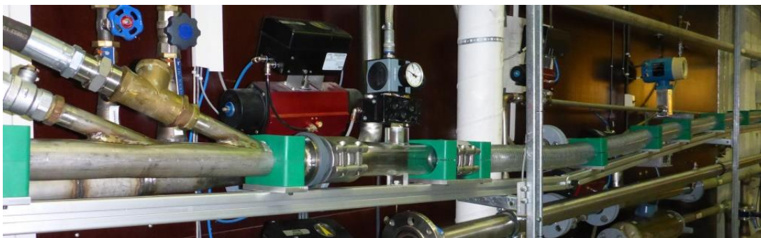
Figure 23: The S-riser nozzle was attached to a downwards inclined rail and connected to a short plexi pipe that was connected to a flexible hose. The construction created a one meter downwards inclined flowline, with a four cm drop. Then the flexible hose was approximately horizontal for 50 cm, before it was inclined upwards again to create the dip geometry outlined in figure 25.
