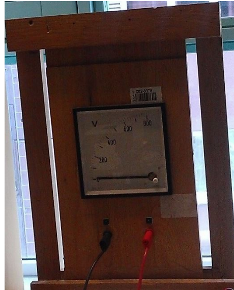
(b) DC voltage side measurement of the converter.
