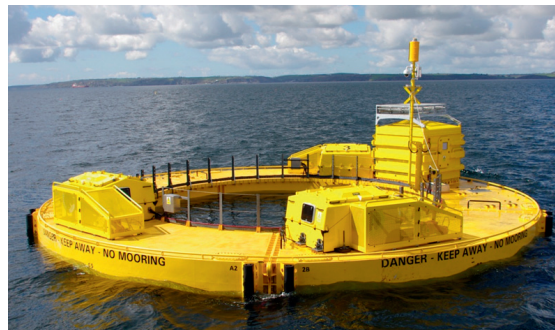
Figure 1. Lifesaver on site outside Falmouth, England.
