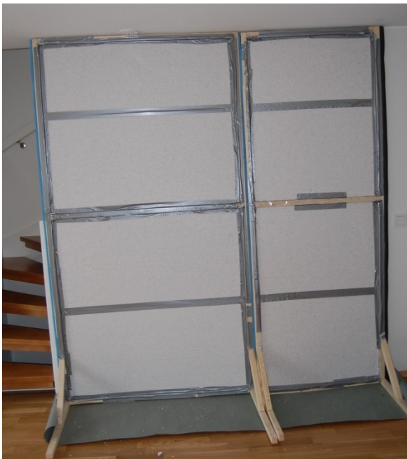
Figure 76: The wall that was built to close of the open staircase.
