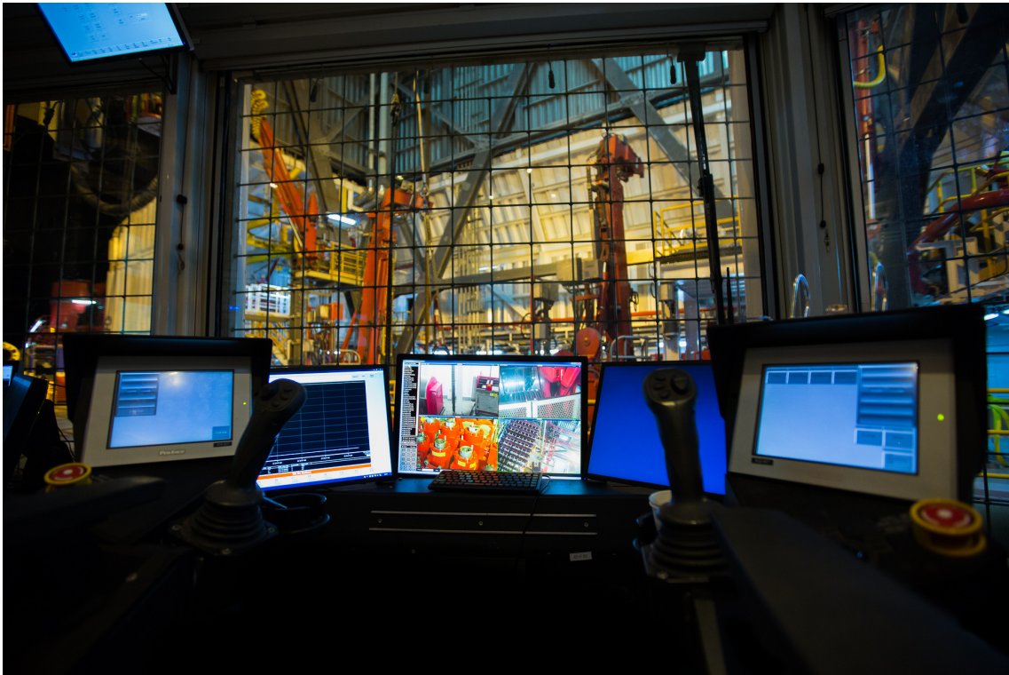
Figure 3.1: Modern driller cabin. Credit: Vegard Haugland, MHWirth AS, Haugland (2015)
