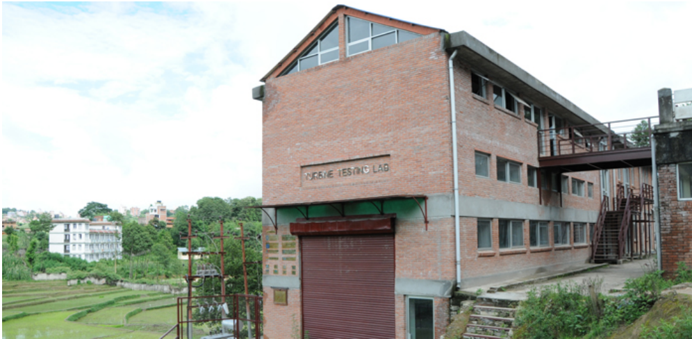
FIGURE 2.3: The Turbine Testing Laboratory plays an important role in the education, research and development of the hydro-power industry in Nepal [8].
