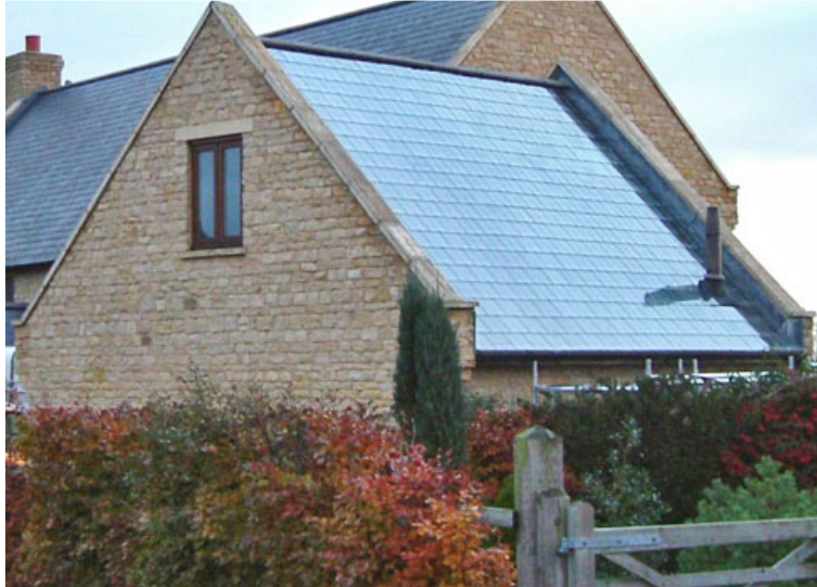
Figure 7-4: In-roof integration of solar collectors [33]
