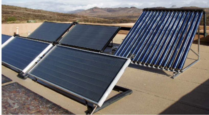
Figure 7-2: Flat on-roof installation with support frames [31]
