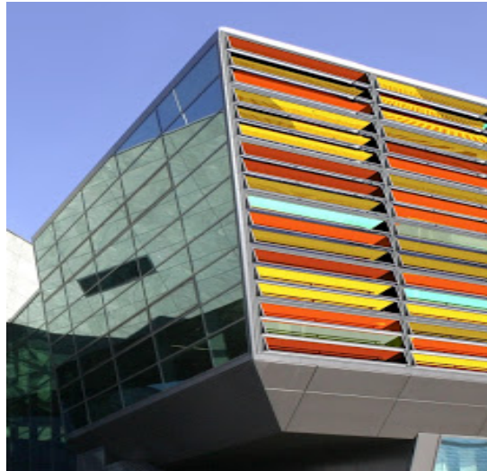
Figure 7-6: Façade integrated solar thermal panels [32]
