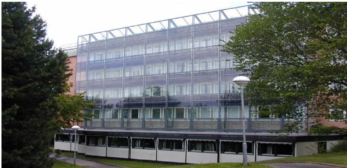
Fig.2.1: O.S. Bragstads plass 2, with BP solar modules in a double façade [20]
