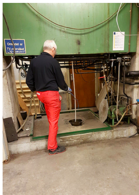
(b) The basement right under the extruder.
