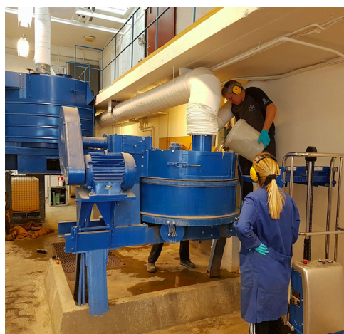
(a) Picture from the mixing of the concrete. At the picture it can be observed water being added into the blender with the aggregate and cement mixture.
