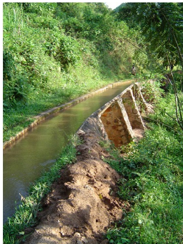
FIGURE 7.10: Open flume of a micro hydropower installation in Rwanda [31]
