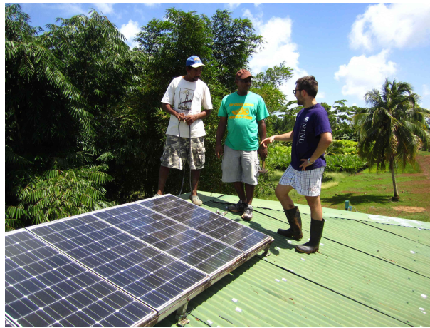
FIGURE 4.8: Installation of PV panels on the roof of the carpenters' house
