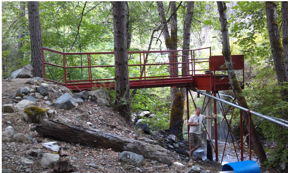
FIGURE 7.8: Installation of LH1kW [30]
