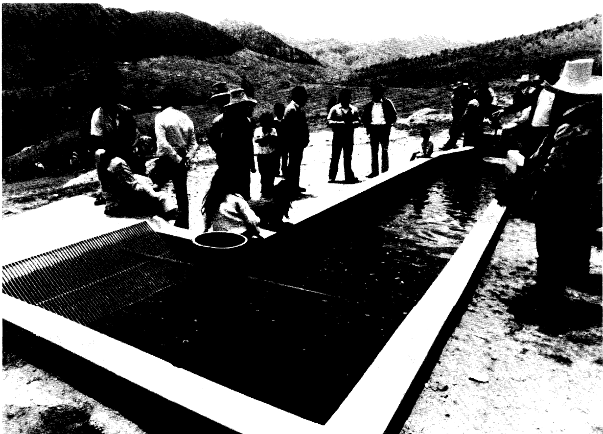
Photo 3.5.3 A pipe plug is used to sluice the forebay silt tank with help from the flush gate at the entry. (Peru)
