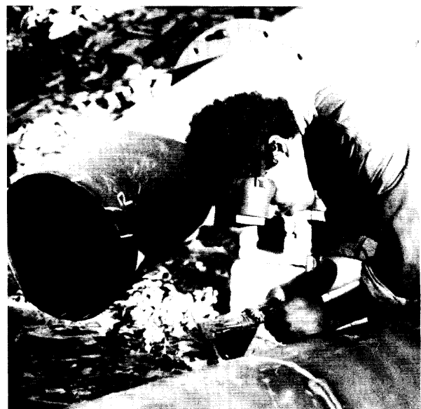
Photo 3.8.3 Steel penstocks can be welded on site if skilled operators are available. (Peru)
