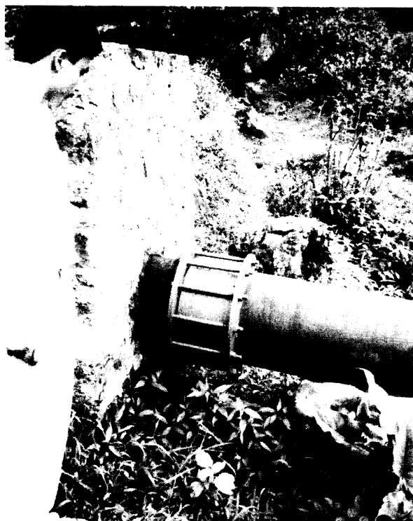
Photo 3.9.1 An expansion joint is best situated just below an anchor block.
