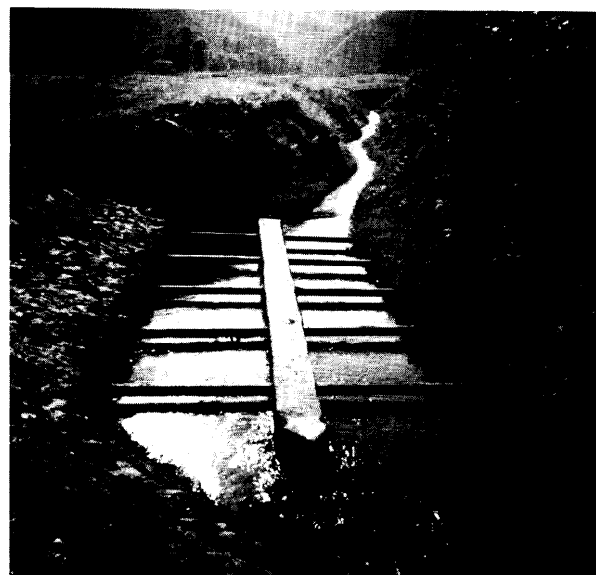
Photo 3.5.1 A partitioned silt basin. (Nepal)
