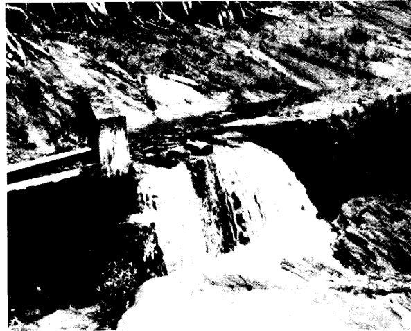
Photo 3.4.1 A block bridge and channel spillway.
