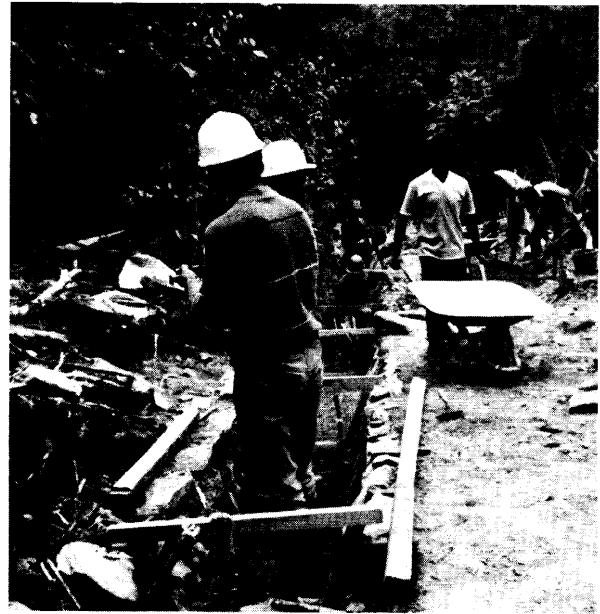
Photo 3.6.2 Wooden formers are very useful when constructing a channel.
