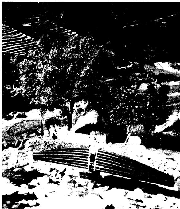
Photo 3.11.1 Plastic pipe (HDPE) being transported by foot in Nepal. Micro-hydro economic decisions are affected strongly by transport costs in some areas.
