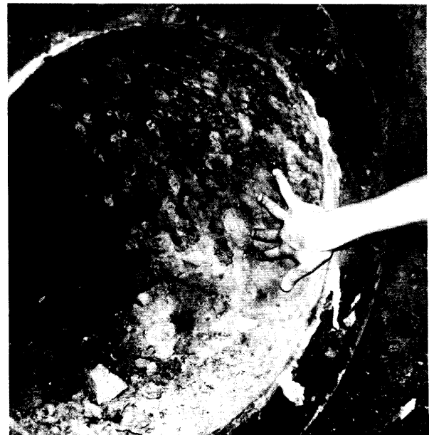
Photo 3.11.5 Corrosion inside a steel penstock. Here the roughness index 'k' can be estimated by observation.
