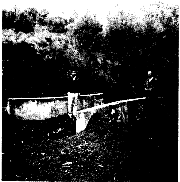
Photo 3.6.3 A channel crossing offers better protection than a culvert
