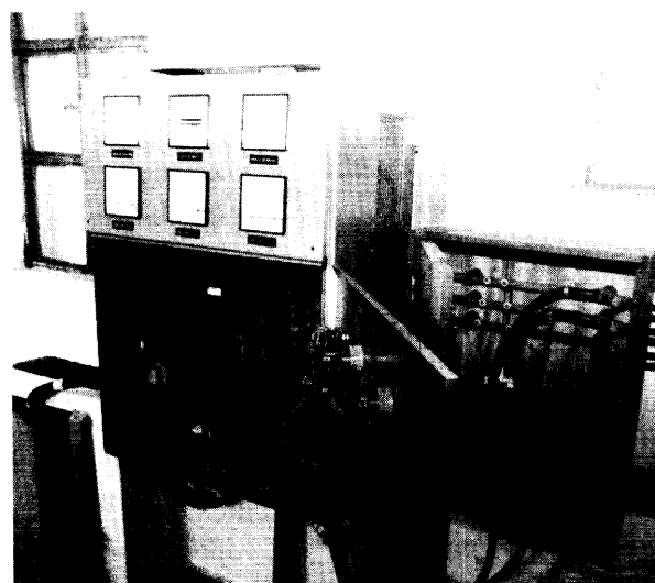
Photo 6.4.1 An electronic load controller (ELC). (Peru)
