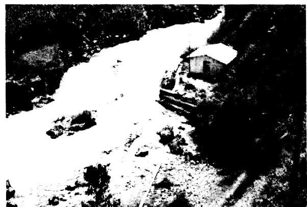
Photo 2.6.2 A powerhouse placed too close to the river.
