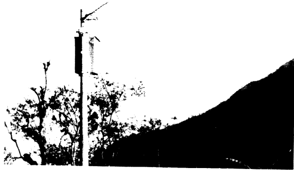
Photo 8.8.2 1 kV to 220 V transformer. (Nepal)
