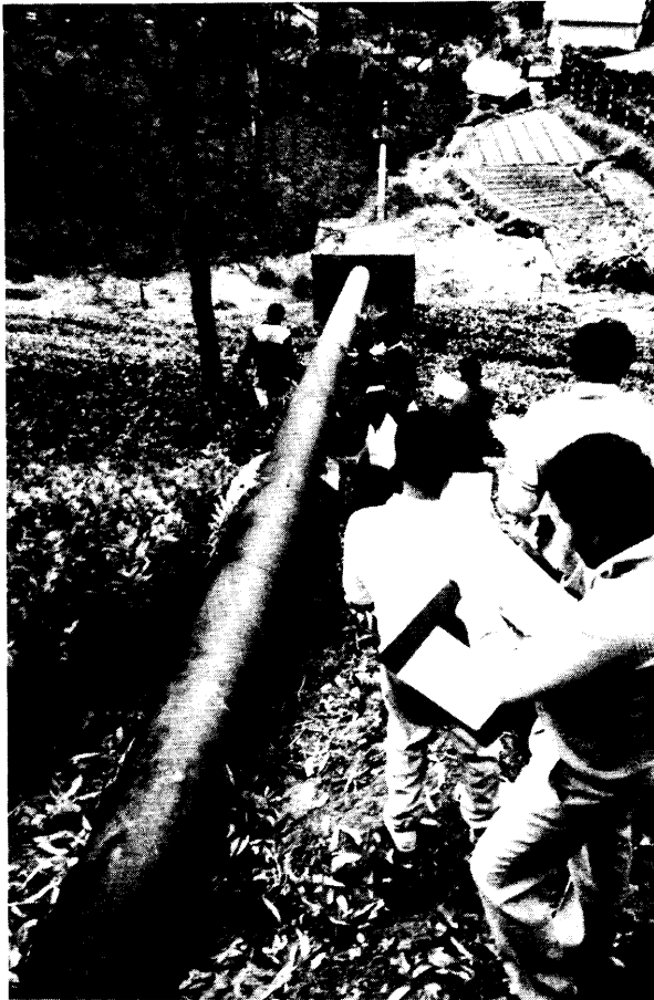
Photo 3.8.2 A mild steel penstock. (Sri Lanka)
