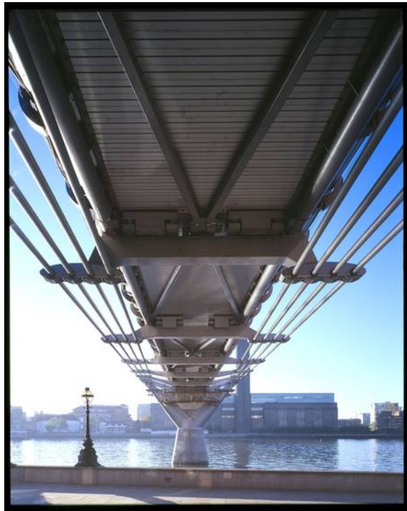
Figure 2.14: TMDs under the Millenium bridge, London. (Gerb, 2018)
