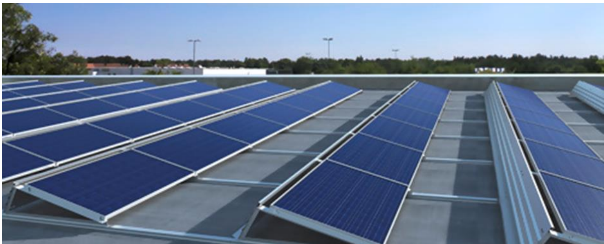
Figure 10 - Illustrates that sloped PV panels need more roof area than that of the actual cells. Depending on the optimum angular, the area needed on the roof will change. (Schueco, 2013)
