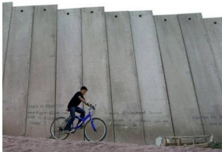
The Security Wall Source: http://mondoweiss.net
