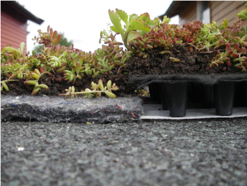
GR used in this study to the left with a substrate layer and a felt mat. Source: Bent Braskerud, VAV
