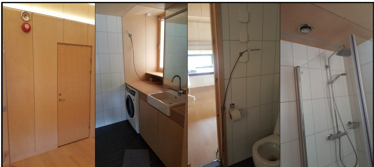
Figure 4.2: Four different views of the test facility at Living lab, Where left image is the entrance to the bathroom, while the other three shows three different angles inside it. The extract valve can be seen in the rightmost image, located above the shower.
